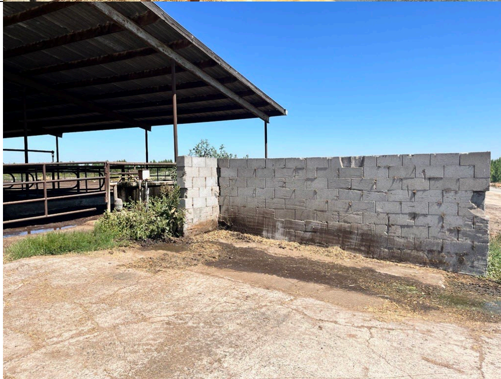
A range of dilapidated structures, useless old walls, and accumulated debris to be removed/disposed
