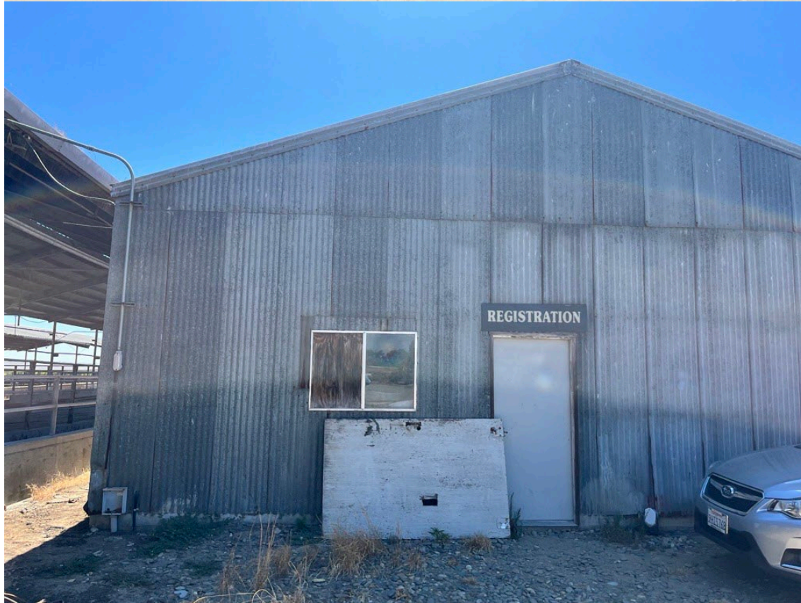
Two buildings to remain/not in scope: milking barn (concrete block bld with attached polebarn) and metal-sided maintenance “registration” shed.
