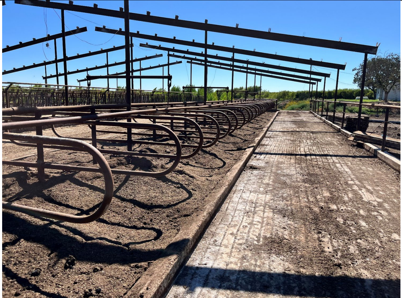
Polebarn 1: Roof and joists already removed. Demo concrete pads, driveway and curbing under this Polebarn 1.
