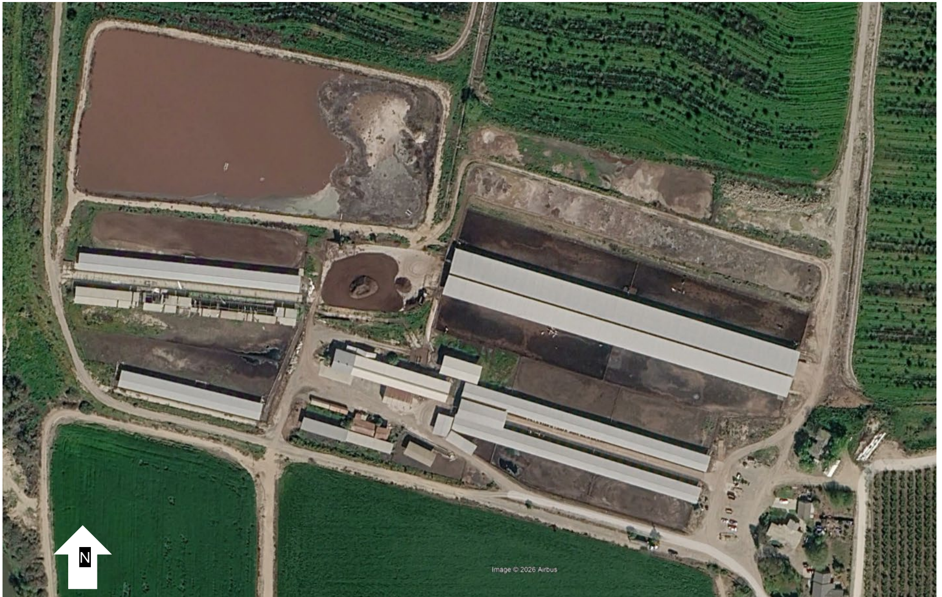
Map 2: Aerial close up of Hidden Valley Dairy site – NOTE THIS IS OUT OF DATE AS SOME PARTIAL DEMOLITION ON POLEBARN HAS ALREADY OCCURRED primarily Roof and roof joist removal.
