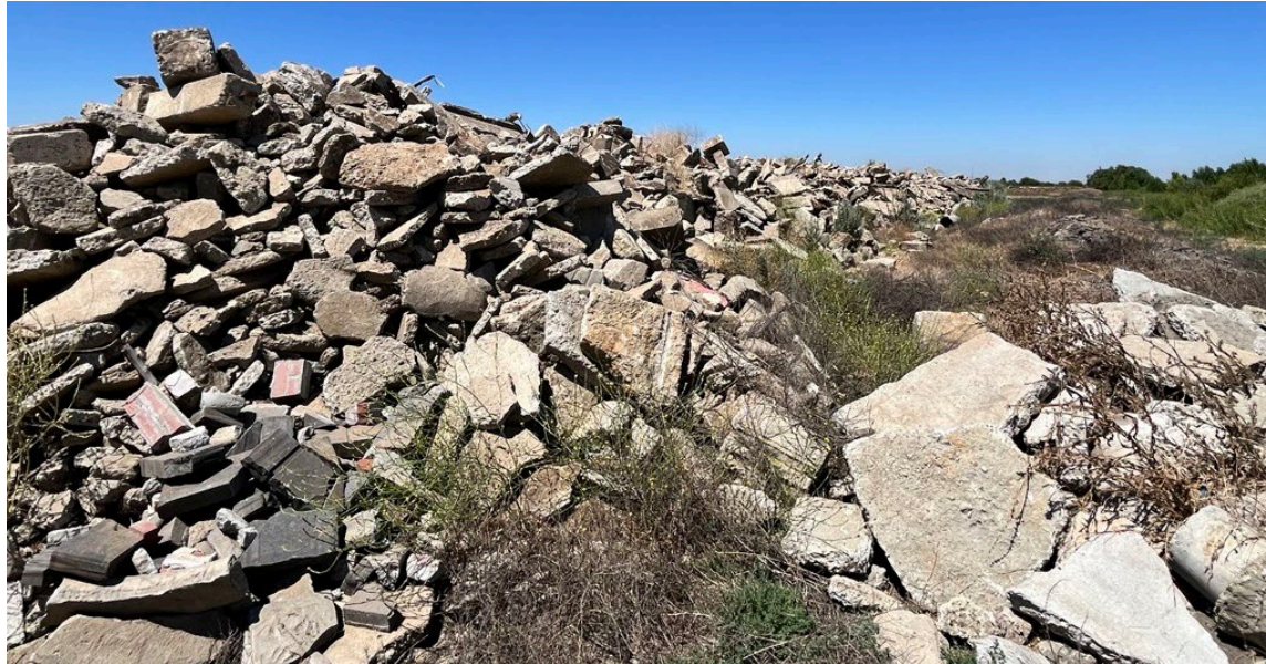
Concrete Stockpile windrow for onsite crushing and/or offhauling removal (~2200 cu yds estimated)
